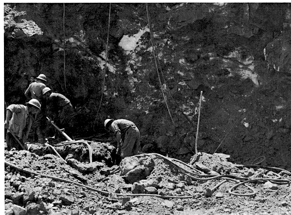
Fig. 5: Excavation at the left side of the rock glacier in the "Combe de Prafleuri" near the resistivity profile G: small crystal size frozen ground, very rich in ice was observed below a thin unfrozen surface layer. Foto taken by W. Fisch 1956.
