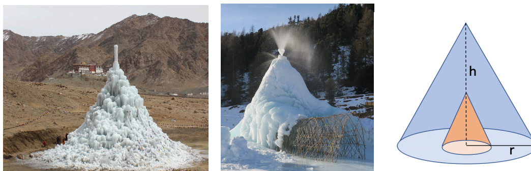
Figure 1. Left: ice stupa in Ladakh, India (c. Sonam Wamchuk). Middle: early growing stage of ice stupa with inner structure in Val Roseg, Switzerland (c. Conradin Clavuot). Right: simple geometrical representation. The stupa can have an inner structure (brown).
