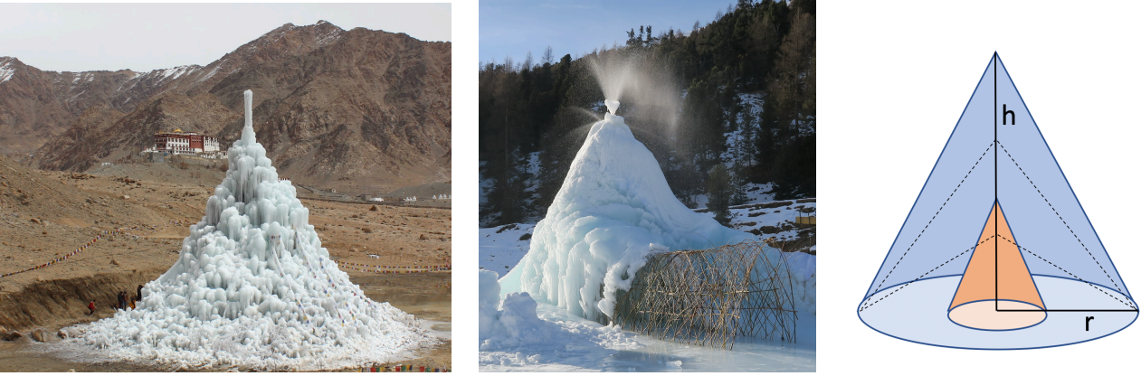
40 Figure 1. Left: ice stupa in Ladakh, India (c. Sonam Wangchuk). Middle: early growing stage of ice stupa with inner structure in Val Roseg, Switzerland (c. Conradin Clavuot). Right: simple geometrical representation. The ice stupa can have an inner structure (brown). The dashed lines illustrate the growth of an ice stupa from a base with a constant radius.
