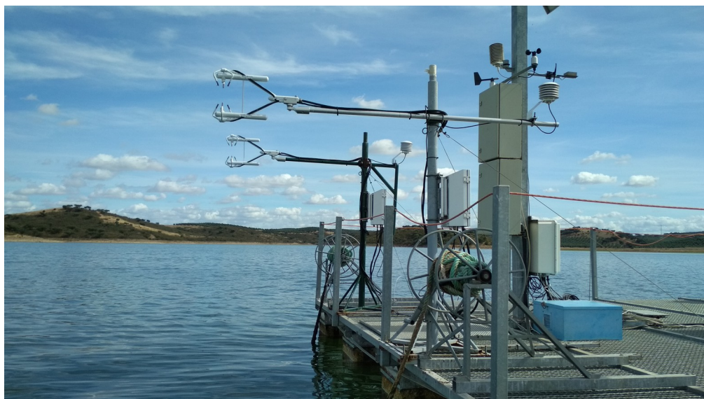
Figure A1: The instruments installed in Alqueva reservoir (Portugal) for the intercalibration. The left instrument belongs to Institute of Earth Sciences, and the instrument on the right belongs to Finnish Meteorological Institute.
