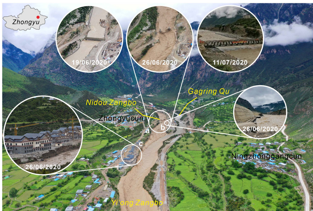
Figure 13. Examples of GLOF damage to downstream infrastructure and buildings at the confluence of Nidou Zangbo and Gagring Qu. Background aerial photo by H. Li taken on 26 June 2020. (a) Comparison of the bridge connecting Zhongyucun and Ningzhonggangcun before, during (photos: H. Li) and after the GLOF (rebuilt, photo: K. Ma). (b) Destroyed roads (photo: H. Li). (c) Affected buildings at risk (photo: H. Li).
