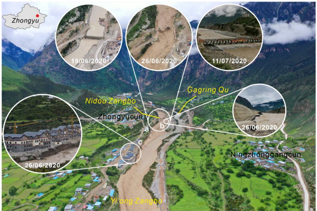
Figure 12. Examples of GLOF damage to downstream infrastructure and buildings at the confluence of Nidou Zangbo and Gagrang Qu. Background aerial photo by H. Li taken on 26 June 2020. (a) Comparison of the bridge connecting Zhongyucun and Ningzhonggangcun before, during (photos: H. Li) and after the GLOF (rebuilt, photo: K. Ma). (b) Destroyed roads (photo: H. Li). (c) Affected buildings at risk (photo: H. Li).
