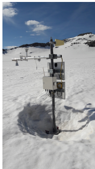
Figure 2: Photo of the mast installation taken in June 2019.
