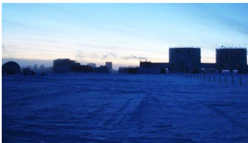
Figure 3: Photograph of Dome C station illustrating the dispersion of the exhaust plume from the electrical power generating plant during conditions with a strong surface temperature inversion. The plume is blown towards the west in the direction of the experimental site. This is a typical situation for a contamination event.
