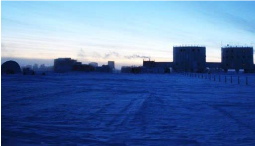
Figure 3: Photograph of Concordia Station illustrating the dispersion of the exhaust plume from the electrical power generating plant during conditions with a strong surface temperature inversion. The plume dissipated toward the west in the direction of the experimental site. This is a typical situation for a contamination event.
