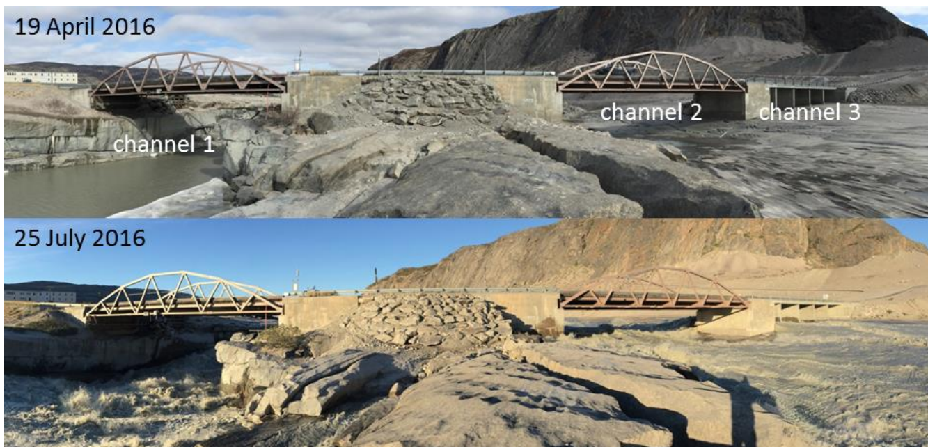
Figure 2: Pictures of the three channels underneath Watson River bridge at low (top) and high discharge (bottom).
