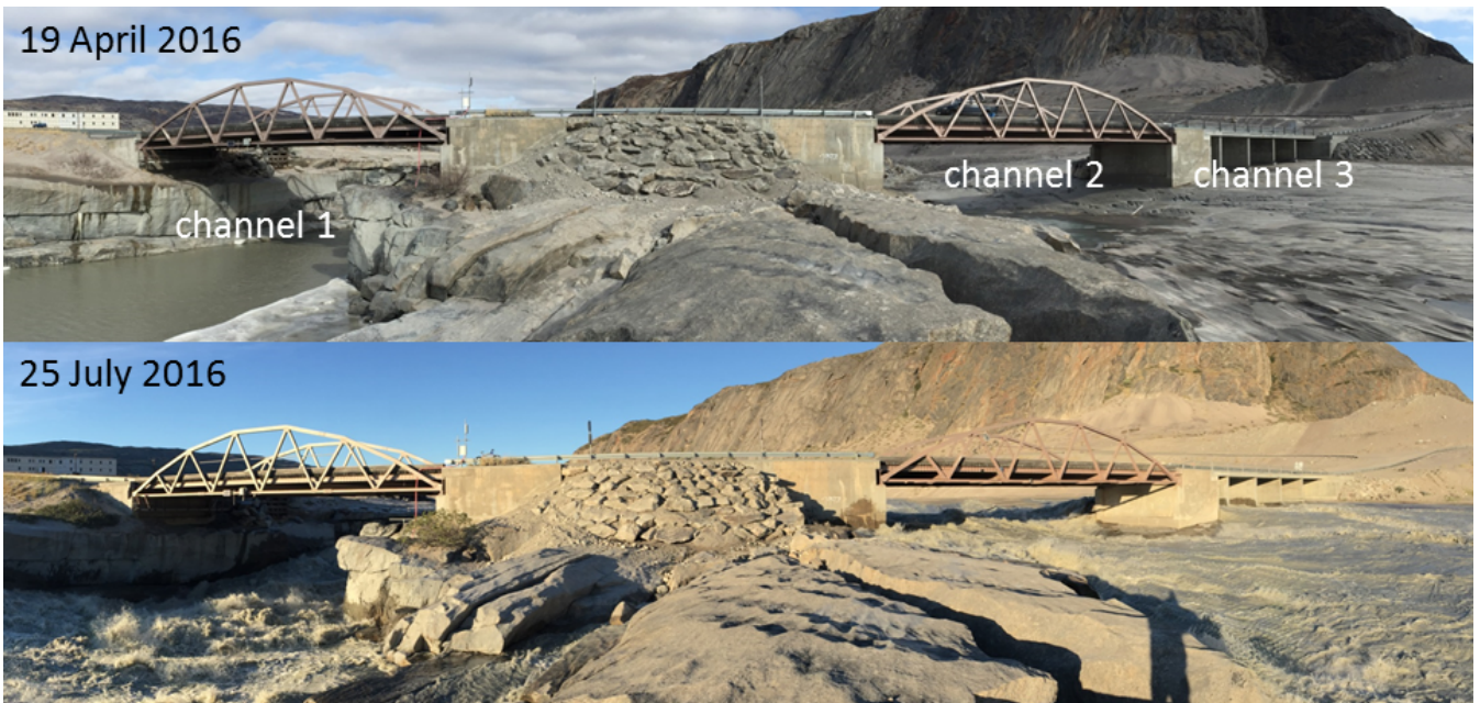
Figure 2: Pictures of the three channels underneath Watson River bridge at low (top) and high discharge (bottom).
