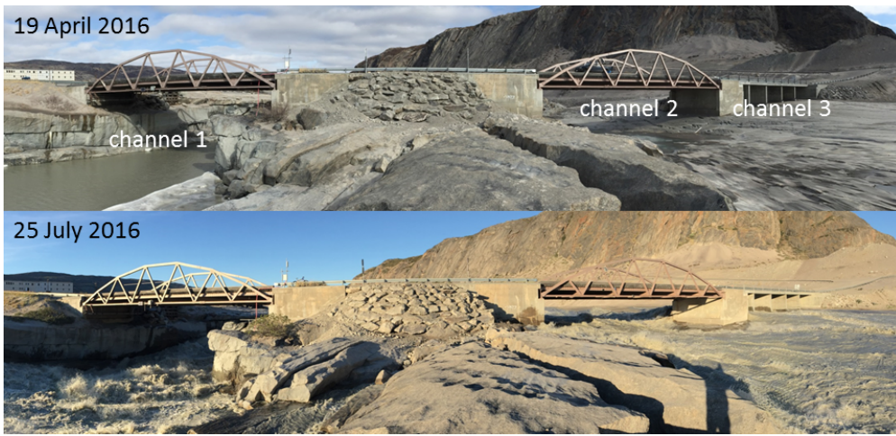
Figure 2: Pictures of the three channels underneath Watson River bridge at low (top) and high discharge (bottom).
