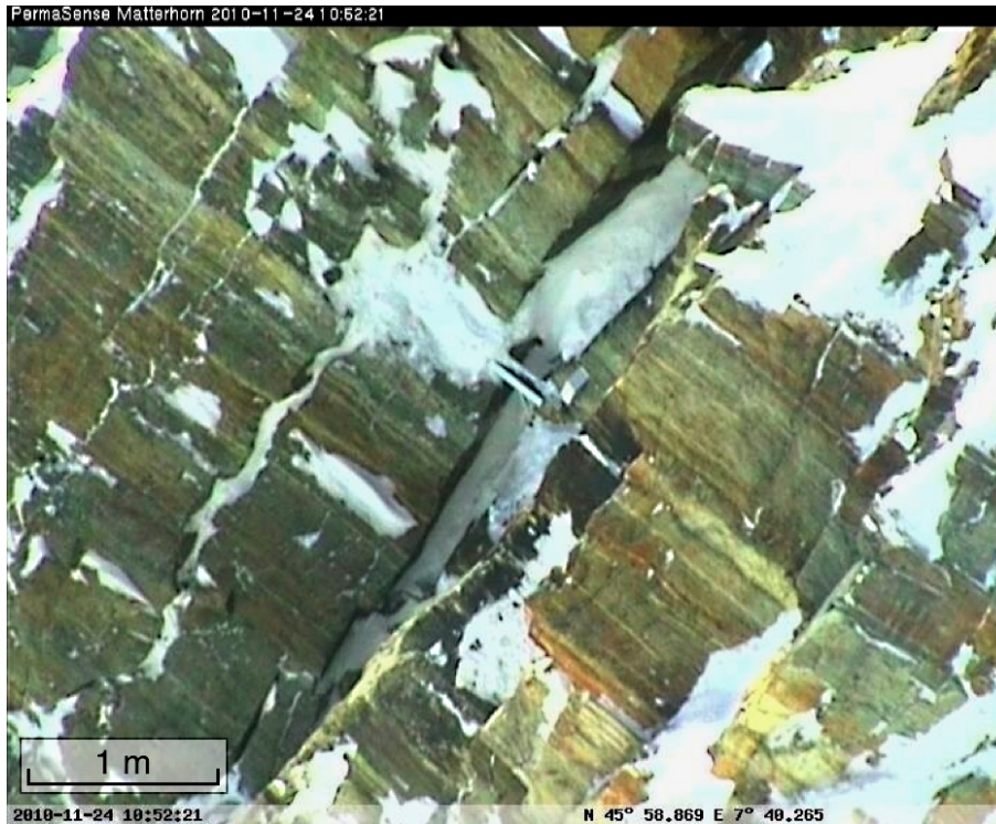
Fig. 4. Fractures with large spacing and opening at Matterhorn Hörnligrat (picture from November 2010). The instrument in the center is a crackmeter, not considered in this article.
